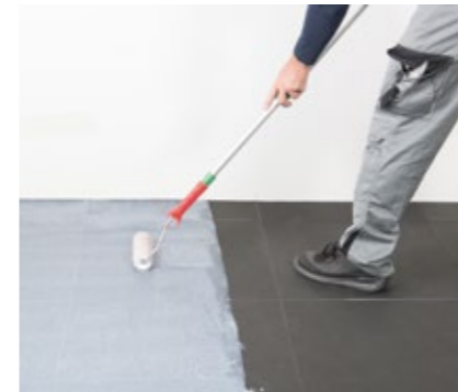
Application of the pressure sensitive adhesive
